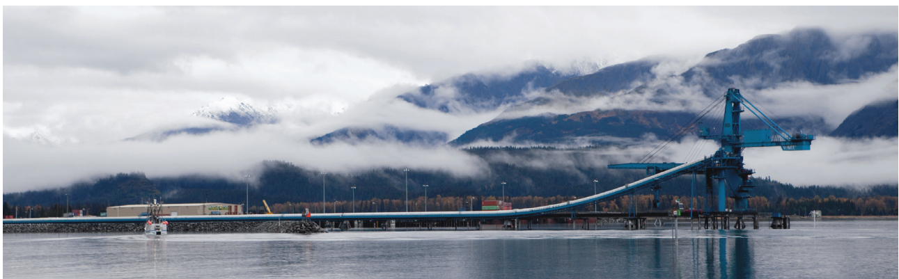
At the Port of Seward in Alaska, Martin completed a conveyor system upgrade for the port’s coal handling operations that has raised throughput by an estimated 20%.
