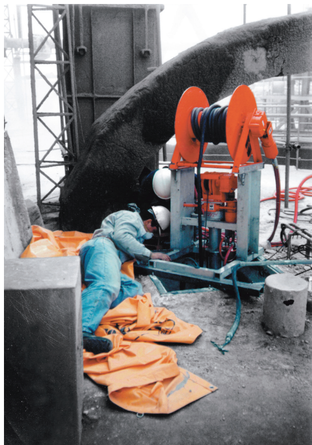
The future lies in providing solutions, not just equipment, particularly in the growing area of outsourced maintenance contracts, such as silo cleaning.
