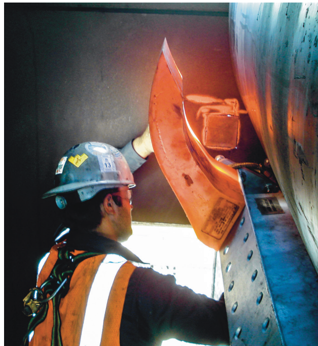
A Martin technician installs a new belt cleaning system as part of a carryback testing programme that was undertaken for a Powder River Basin coal mine. The Martin system used just two cleaners per belt, instead of four.
